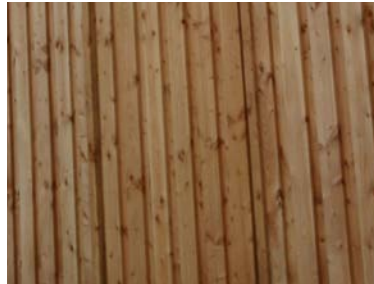
Timber wall without paint
