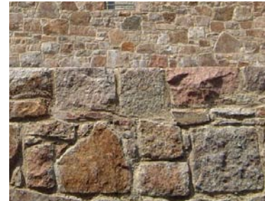
French granite could be used as ground floor wall material and for paving.
