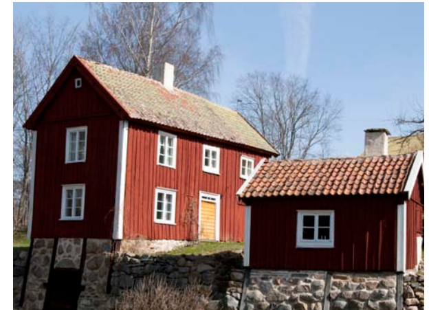
Walls painted with Swedish Falu rödfärg.
