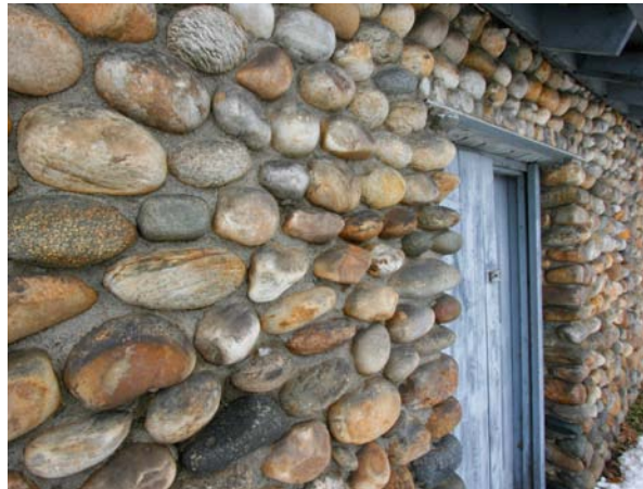
Local river stones used as a facade material
