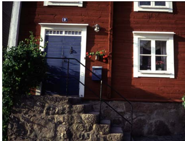
Granite masonry base with red painted timber above.
