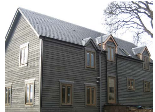
Vertical windows on front and side elevations.
